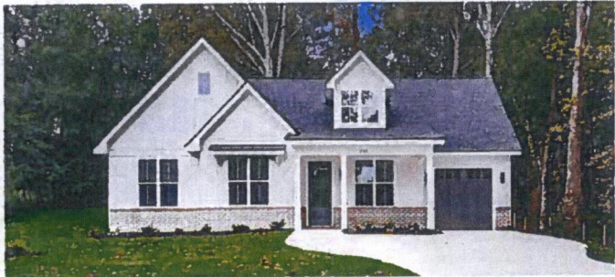
Farmhouse Elevation Powder Springs Home, Completed 2025
